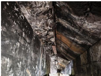
Figure 5. Damage to the Bridge Deck Slab
