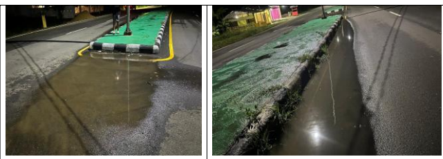
Figure 2. Surface ponding on flexible pavement
