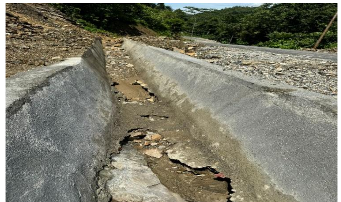
Figure 1. Scouring of drainage channels
