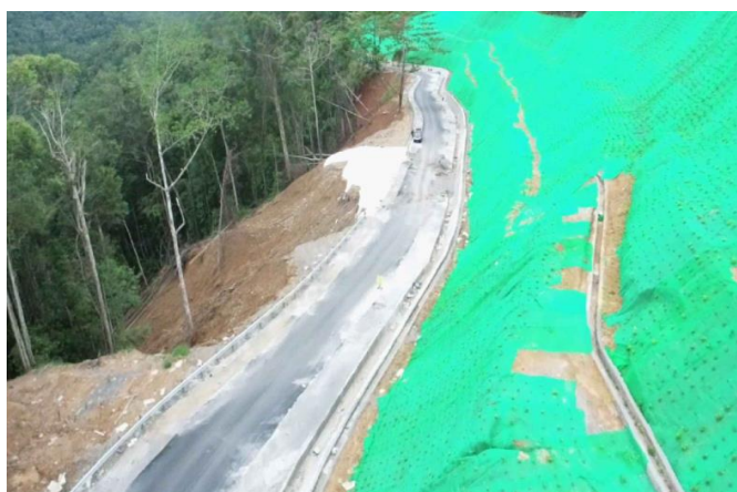
Figure 3. Existing condition of STA 34+990 – 35+020
