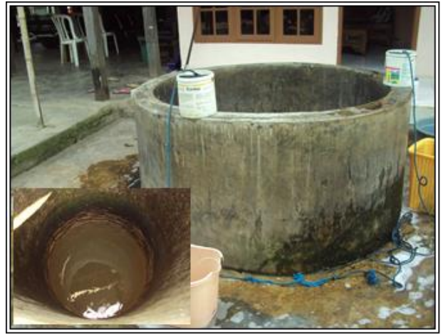
Figure 5 Photograph view of the S05 Water Sampling Well in the Lemmobeng area, photographed towards N120°E.
