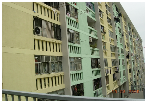
Figure 8. View of façade with typical balconies
