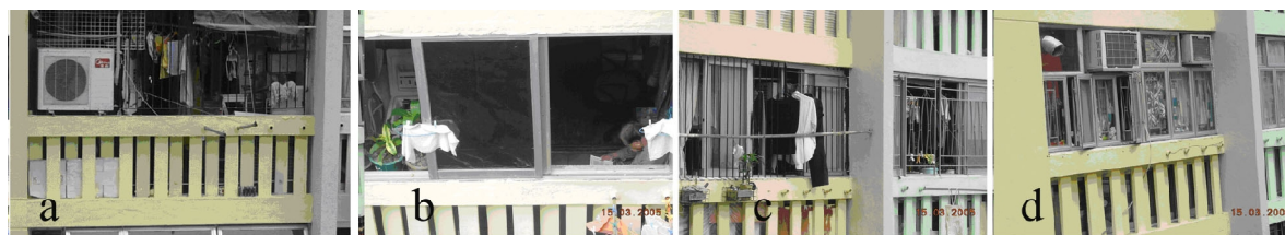
Figure 7. Changes in balconies: a) without glazing, b) utility space, c) & d) as additional rooms.
