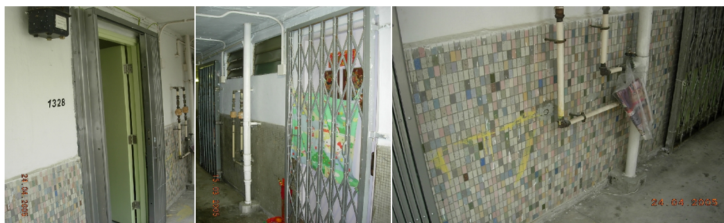
Figure 9. Change in front doors a) the time of delivery b) modified with curtains and altar. Materials outside the front door c) wall: small tiles, and floor: neat cement
