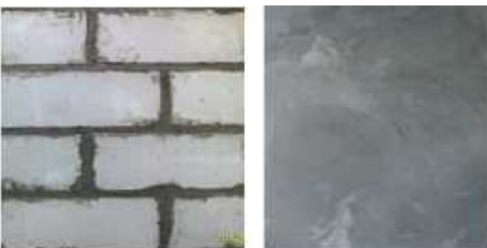
Fig. 7 Wall specimen of lightweight brick, before and after plastering
