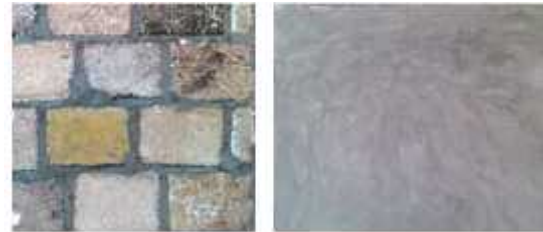
Fig. 8 Wall specimen of local limestone brick, before and after plastering
