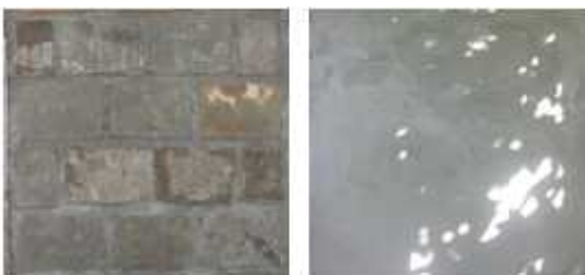
Fig. 6 Wall specimen of epoxy-sawdust brick, before and after plastering
